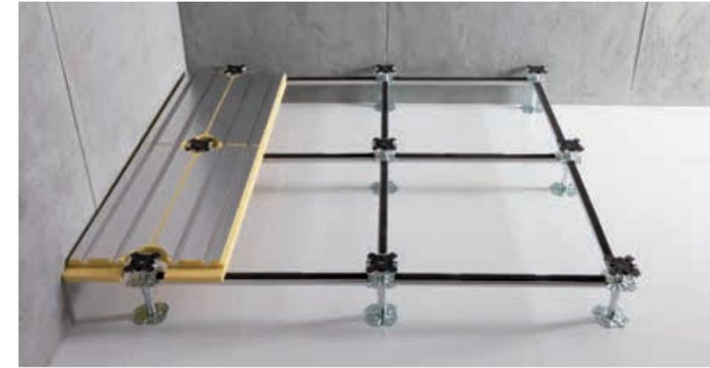
**3/** Complete the laying of "active" panels on all the pedestal rows.
